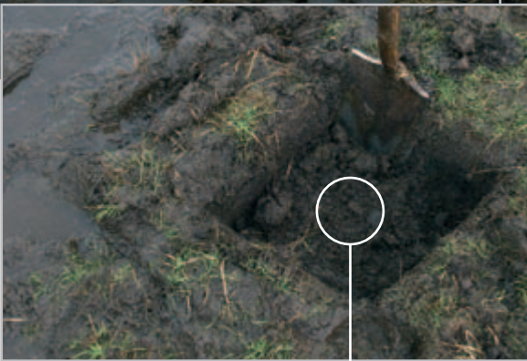
Dry subsoil with poor soil structure
